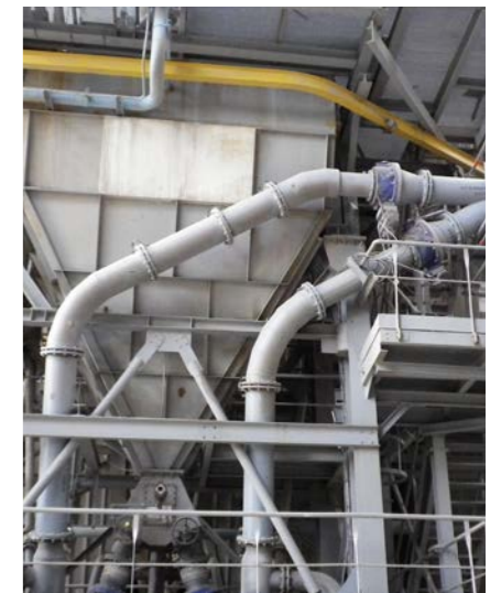
Pneumatic KALOCER transfer line with moulded components for conveying alternative fuel (demolition wood with sand particles) to a furnace, cross-section 203 mm
