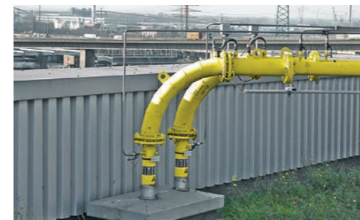
KALDETECT in a German waste incineration plant
