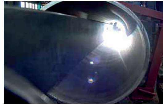
Automatic welding machine for lining the interior of a pipe
