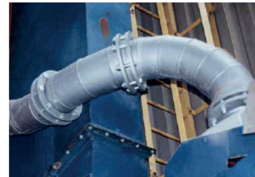
ABRESIST pipes and pipe bends protect against abrasion and corrosion
