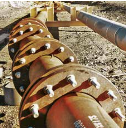
Extended service life of plant components
