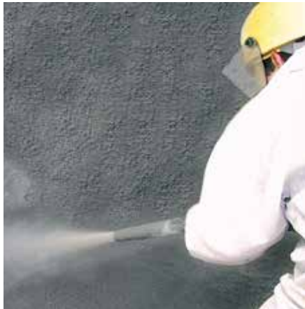
Kalenborn service solves wear problems on site
