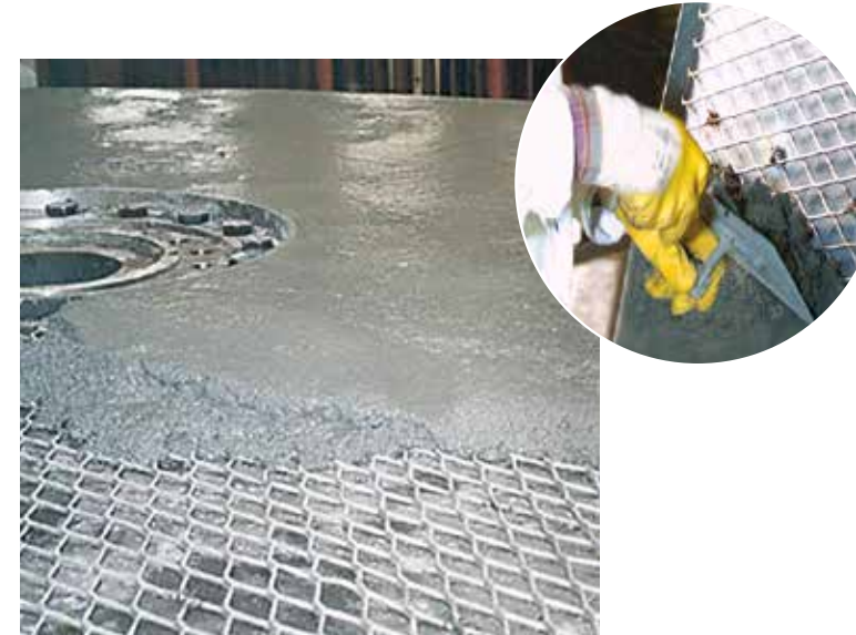
Separators are frequently protected by KALMETALL hard overlay welding or by KALCRET hard compound (pictures) installed without joints.
