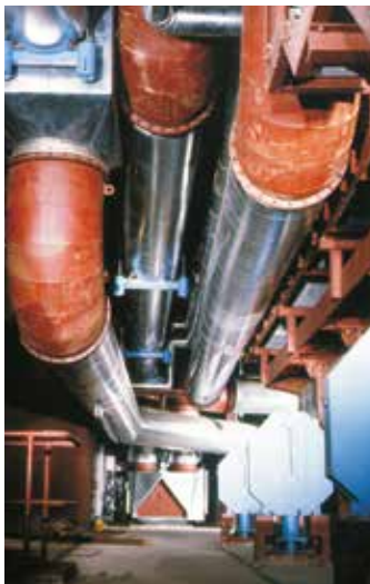
A typical application in power plants is pulverized fuel piping.
