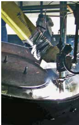
Rebuilding a grinding table with KALMETALL W100.
