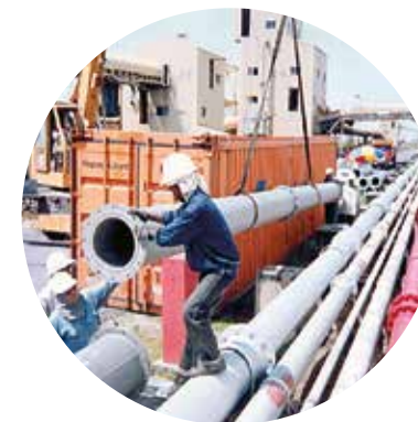
Installation of wet ash pipes in Malaysia (350 mm diameter).
