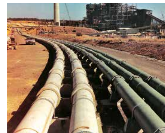
Wet ash pipe in North America; the pipes are flanged together.
