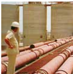
ABRESIST fused cast basalt is the accepted standard for piping in wet ash pipe systems all over the world. The picture shows a plant in India.
