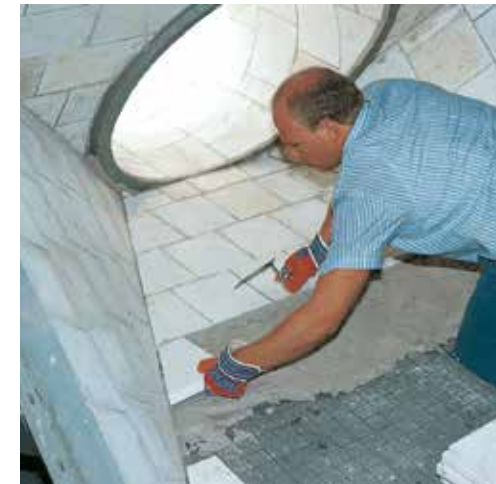
Collecting hopper being part of sintered material dust collection at 400° C / 752° F: effectively protected with KALCOR zirconium corundum
