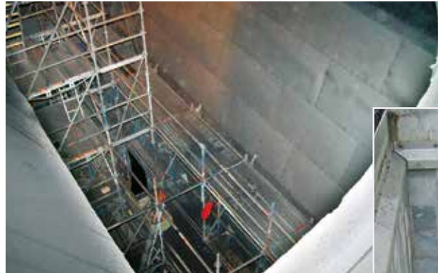
A trouble-free material flow is ensured in coal bunkers by the use of KALEN slide promotion plastics
