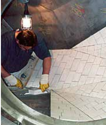
Octagonal hopper with KALOCER lining; for optimal adaptation the 50 mm thick shaped elements have been cut three-dimensionally
