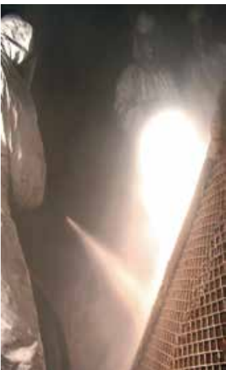
Short lining times for a whirler are achieved with a combined lining of hard compound KALCRET BTS and zirconium corundum KALCOR. The high application rate of KALCRET BTS is 5 m 2 /h
