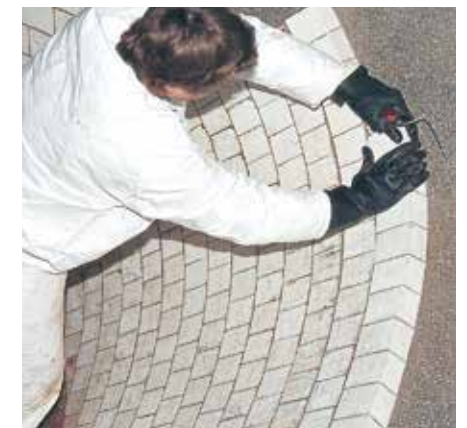
Kalenborn service solves wear problems on site
