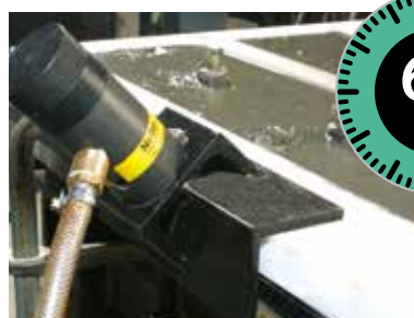
4. Use external vibrator for compacting
