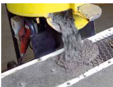
3. Carefully fill formwork
