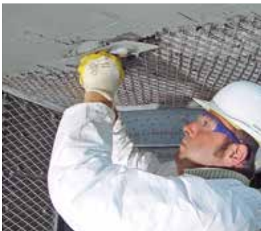
1. Overhead working is feasible without problem
