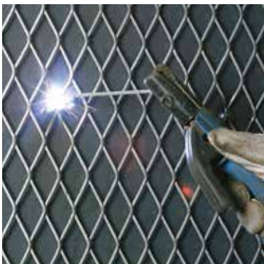
Welding the wire mesh to the surface: spacing approx. 250 mm / 9.8 inches
