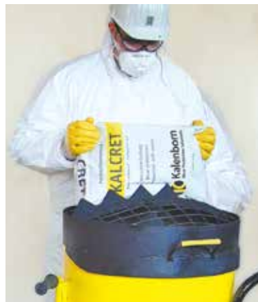
Material feeding into the forced circulation mixer
