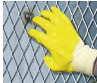
Stiff and rigid fastening – distance to the wall to be lined: about 5 mm / 0.19 inches
