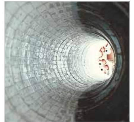
Pipe bend with ABRESIST and KALOCER combined lining
