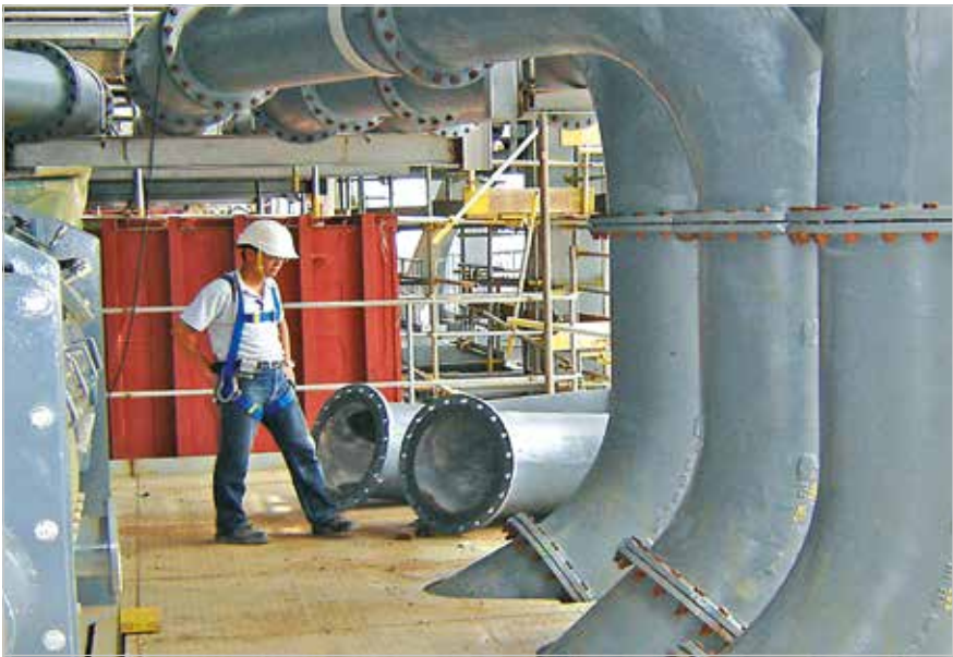
Typical applications of KALCAST hard casting are pipe systems; here a pulverized coal pipe of a power station in South East Asia
