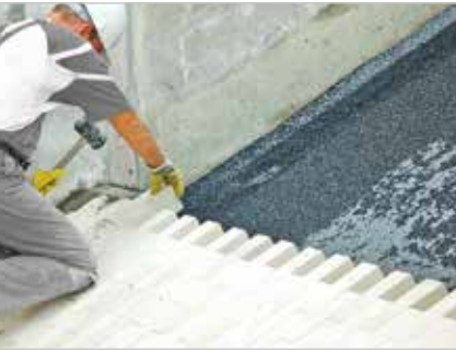
High temperature KALCERAM chute in a coking plant provides good sliding properties even at high temperatures
