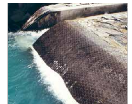
Irrigation weir protected by ABRESIST
