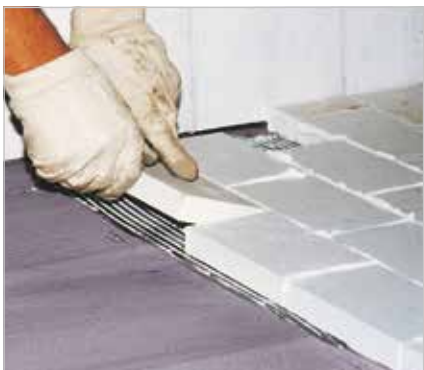
Lining and fixing with synthetic resin putties
