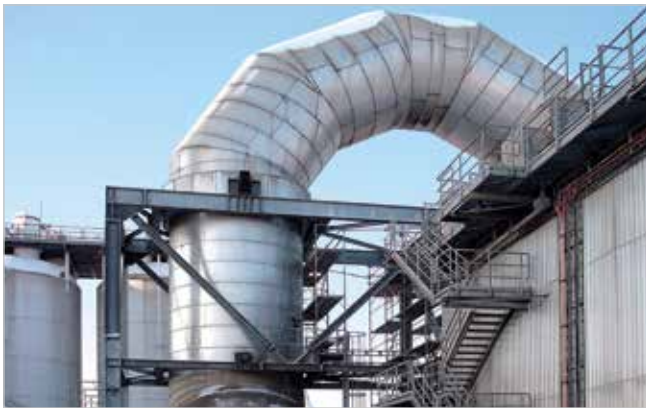
Clinker dust line in cement plant
