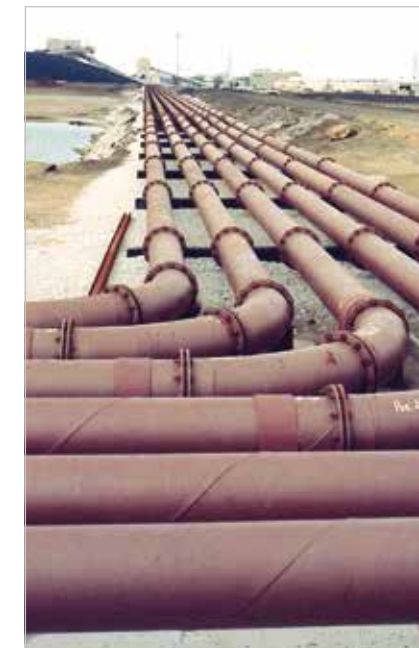
Worldwide ash removal pipes lined with ABRESIST reach lifetimes of more than 30 years. This US power plant operates more than 10,000 meters of 294 mm ID pipes.
