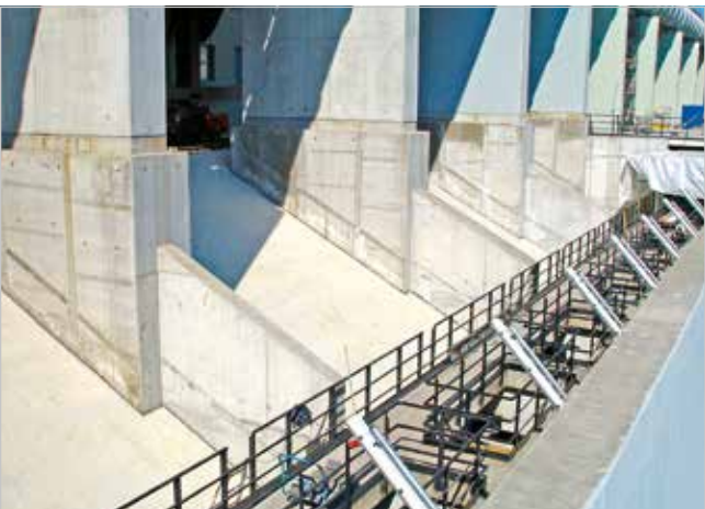
Coke wharf protected with KALCERAM K on the sliding surface, with KALSICA N in the zone of high wear and with KALCAST in the area of impact stress
