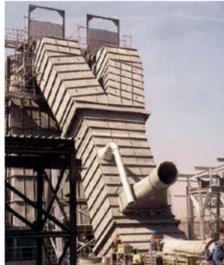
Cooler waste gas pipe lined with KALCRET BNY hard compound
