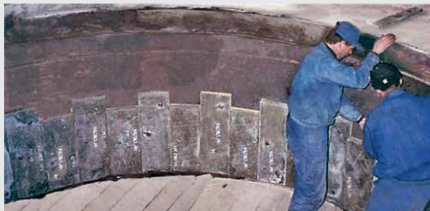
Protection of raw meal pipes against abrasive wear with hard compound KALCRET, lining thickness 25 - 40 mm, operating temperature 200 °C / 392 °F
