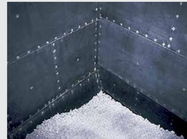
Limestone bunker with slide promoting lining made of KALEN 1006
