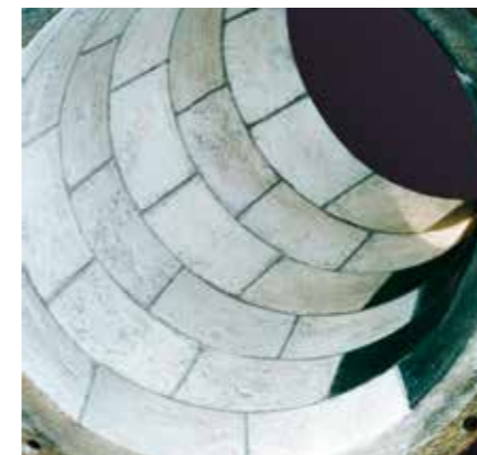
Material combinations are an advantage for pipes of larger diameter. Here ABRESIST fused cast basalt has been combined with KALCOR zirconium corundum.
