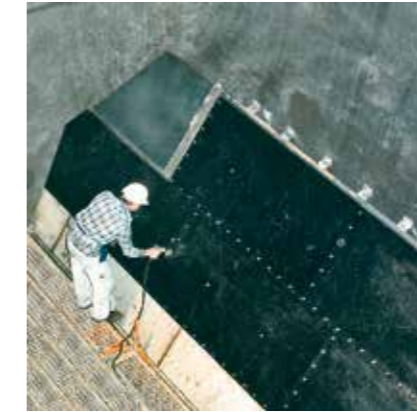
Large bunkers are efficiently and reliably lined with KALEN slide promotion plastics.
