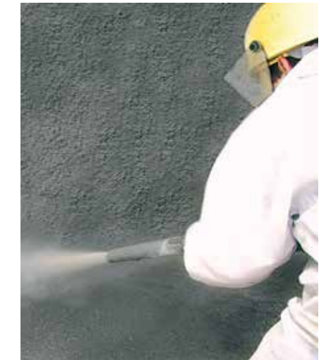
Kalenborn service solves wear problems on site
