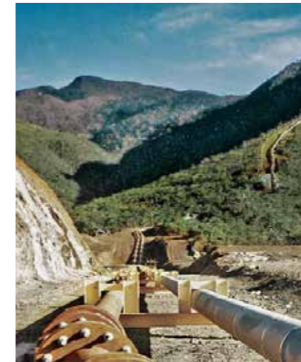
Extended service life of plant components
