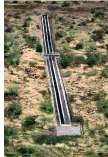
Hydraulic drop chutes can be operated over long periods provided they have been appropriately lined. ABRESIST fused cast basalt is often the preferred choice.
