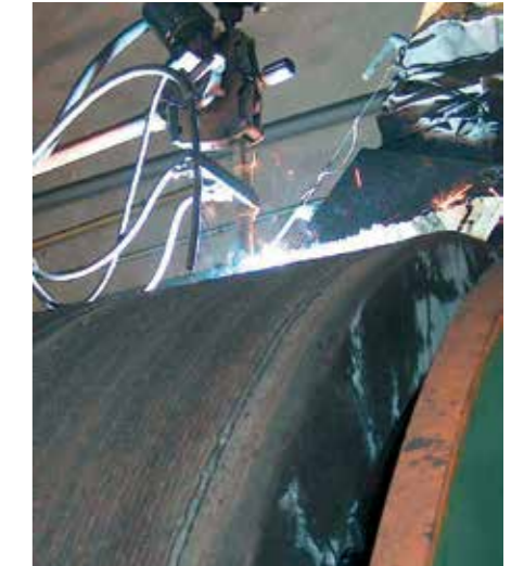
Kalenborn field service solves wear problems on site
