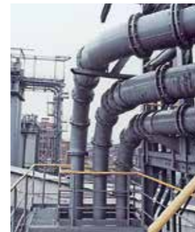
Fly ash pipes are among the plant components that are particularly endangered by wear. Kalenborn offers a variety of materials to ensure optimal service lifetimes: ABRESIST fused cast basalt, KALCOR zirconium corundum and KALOCER high alumina ceramics.
