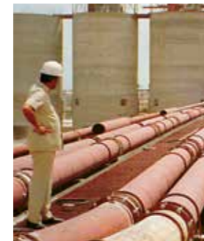
ABRESIST fused cast basalt is the accepted standard for piping in wet ash pipe systems all over the world. The picture shows a plant in India.
