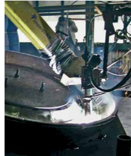
Rebuilding a grinding table with KALMETALL W100.
