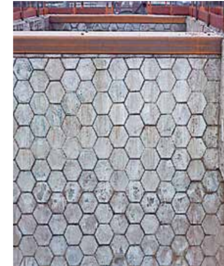
Extended service life of plant components
