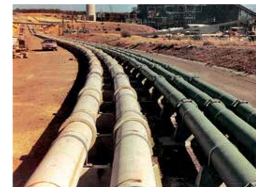
Wet ash pipe in North America; the pipes are flanged together.
