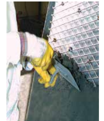
Separators are frequently protected by KALMETALL hard overlay welding or by KALCRET hard compound (pictures) installed without joints.
