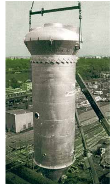
Dust collection cyclones for blast furnaces are effectively protected with combined linings
