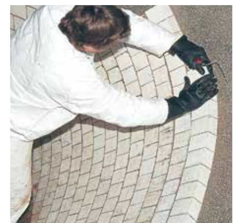
Kalenborn service solves wear problems on site
