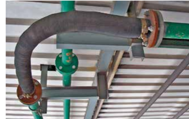
KALFLEX pipe bends in practical operation; here shown as flexible connection between rigid connection points
