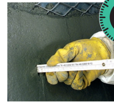
4. Check layer thickness and equalize it, if necessary
