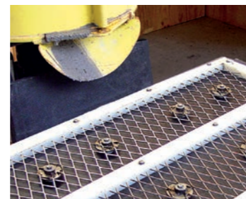
Prepare formwork, attach reinforcement system
