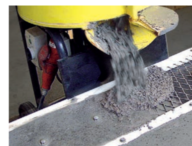
3. Carefully fill formwork
