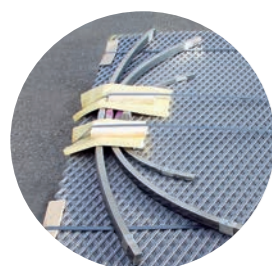
Wire mesh including welding equipment and electrodes, if required
