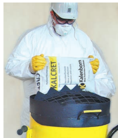
Material feeding into the forced circulation mixer
