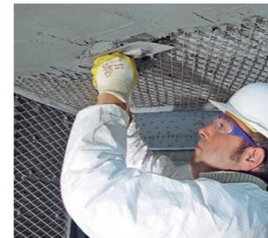
1. Overhead working is feasible without problem
