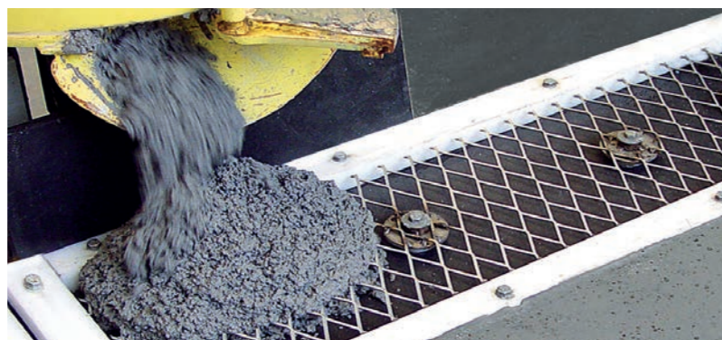
The compound should have a plastic consistency
