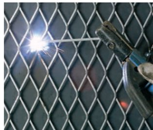
Welding the wire mesh to the surface: spacing approx. 250 mm / 9.8 inches
