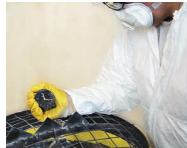
Mix for 4-8 minutes and check result
