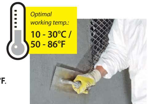
After spraying, easy to make smooth
