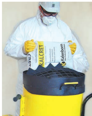
Material feeding into the forced circulation mixer
