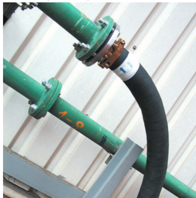
Wear-protected flexible hoses for rapid, simple and inexpensive installation
