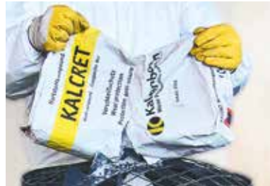
Empty the bag of KALCRET hard compound in the mixer
