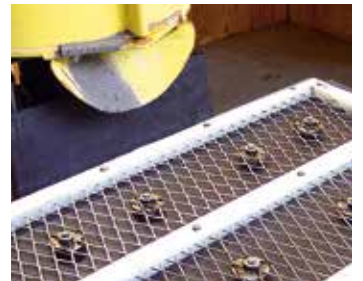
Prepare formwork, attach reinforcement system
