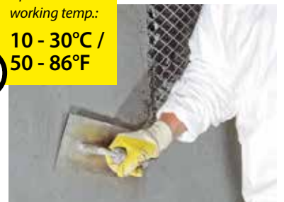
After spraying, easy to make smooth
