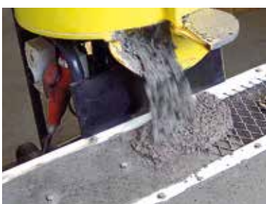
3. Carefully fill formwork
