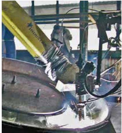
Kalenborn Service solves wear problems on site
